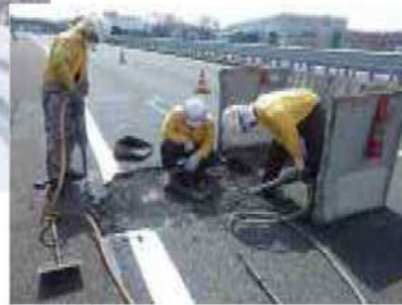
Road Surface Maintenance
