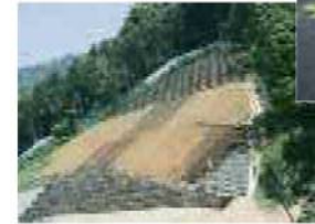
Restoring Works at Hachiiji Junction, the Ken-O Expressway (May 2000)
