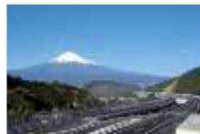
The Opening of E1A (the Shin Tomei Expressway)
