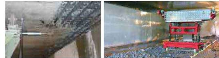
Works at Narrow Places
