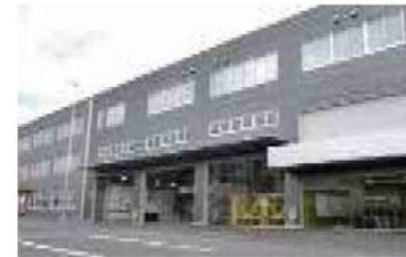
Technical Training Center (Exterior)
