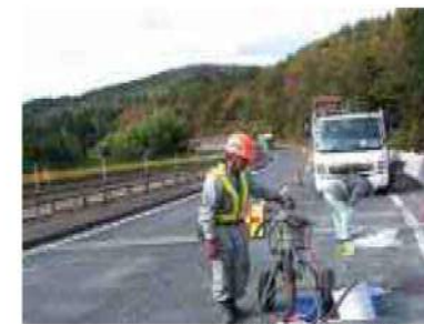
Works from Pavement Surface
