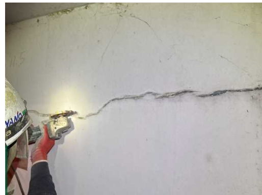
橋梁のひび割れ補修
