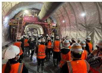
(工事現場の視察)
