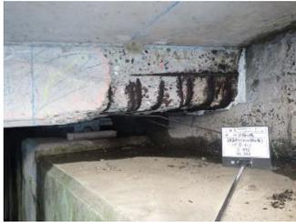
(判定区分Ⅲ：桁端部塩害劣化の補修前)
