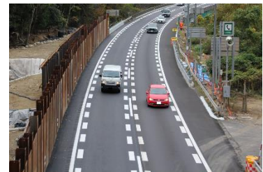
(2車線確保状況)
