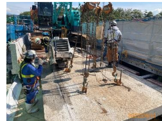
(橋梁床版取替)
