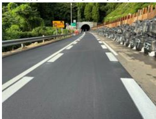
(1車線確保状況)
