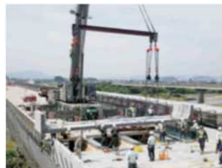
(橋梁床版取替)
