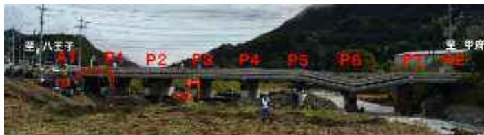
(国交省HP/法雲寺橋被災状況)
