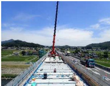
[floor slab replacement]
