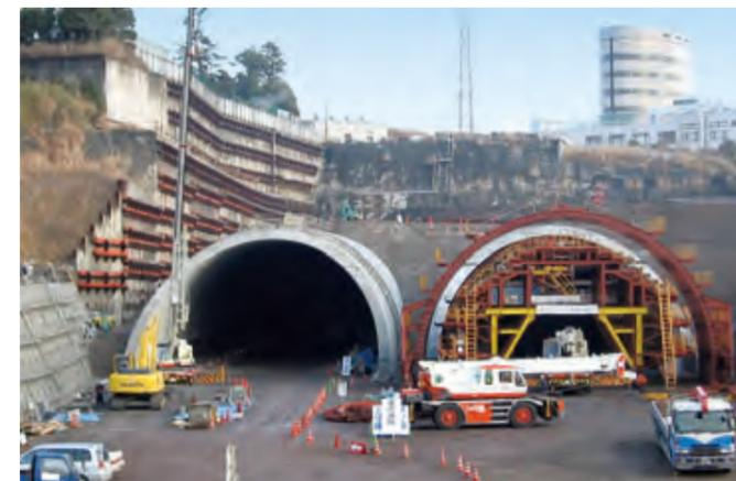
■ Once the tunnel structure is completed, the excavated soil is backfilled to restore the terrain to its original profile, minimizing the tunnel's impact on adjacent residential areas.
