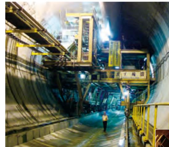
■ The Hida Tunnel is 10.7 kilometers long, with an overburden of 1,000 meters of rock. Since this configuration precluded the placement of vertical ventilation shafts, we employed a longitudinal ventilation system beneath the roadway surface and another ventilation tunnel along the main tunnel.
