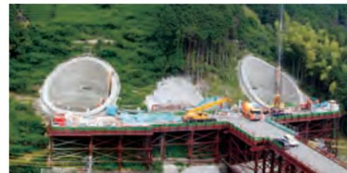
Heavy machinery like the 35-ton dump truck and backhoe with a 5 or 12m<sup>3</sup> bucket, shown below working on the Shin Tomei Expressway, enables rapid construction on large-scale earthwork.
