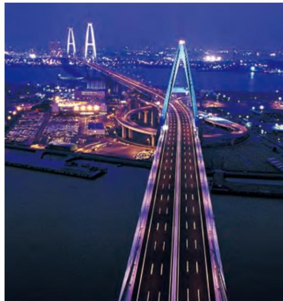
■ Three consecutive cable-stayed bridges on the Ise-Wangan Expressway were constructed in Nagoya's port zone. The bridge sections are 758 meters, 1,170 meters and 700 meters long, respectively, and form a three-lane expressway. These large-scale bridges demonstrate our advanced capabilities.
