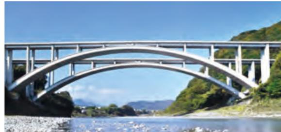
■ This highly engineered bridge (The Shin Fujigawa Bridge) is a steel-concrete composite structure. The arch and vertical members are made of concrete to maintain superior compression characteristics. In contrast, the top girders are made of steel to achieve a lightweight bridge structure. The weight and cost are approximately 40% and 20% less than an ordinary concrete arch bridge respectively.
