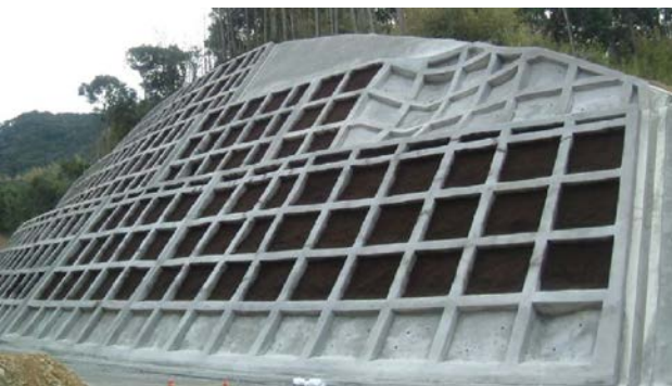
(吹付のり砕工)
