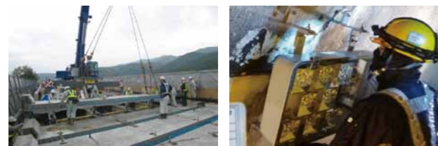
橋梁の床版取換え
