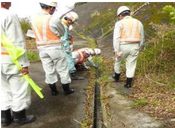
(切土のり面の変状を確認)
